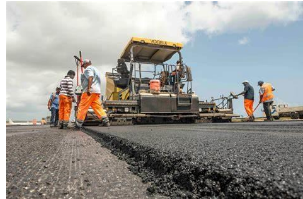
Road construction, NSW
