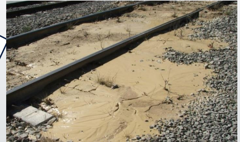
Mud pumping in field (Indraratna et al.,2020)
